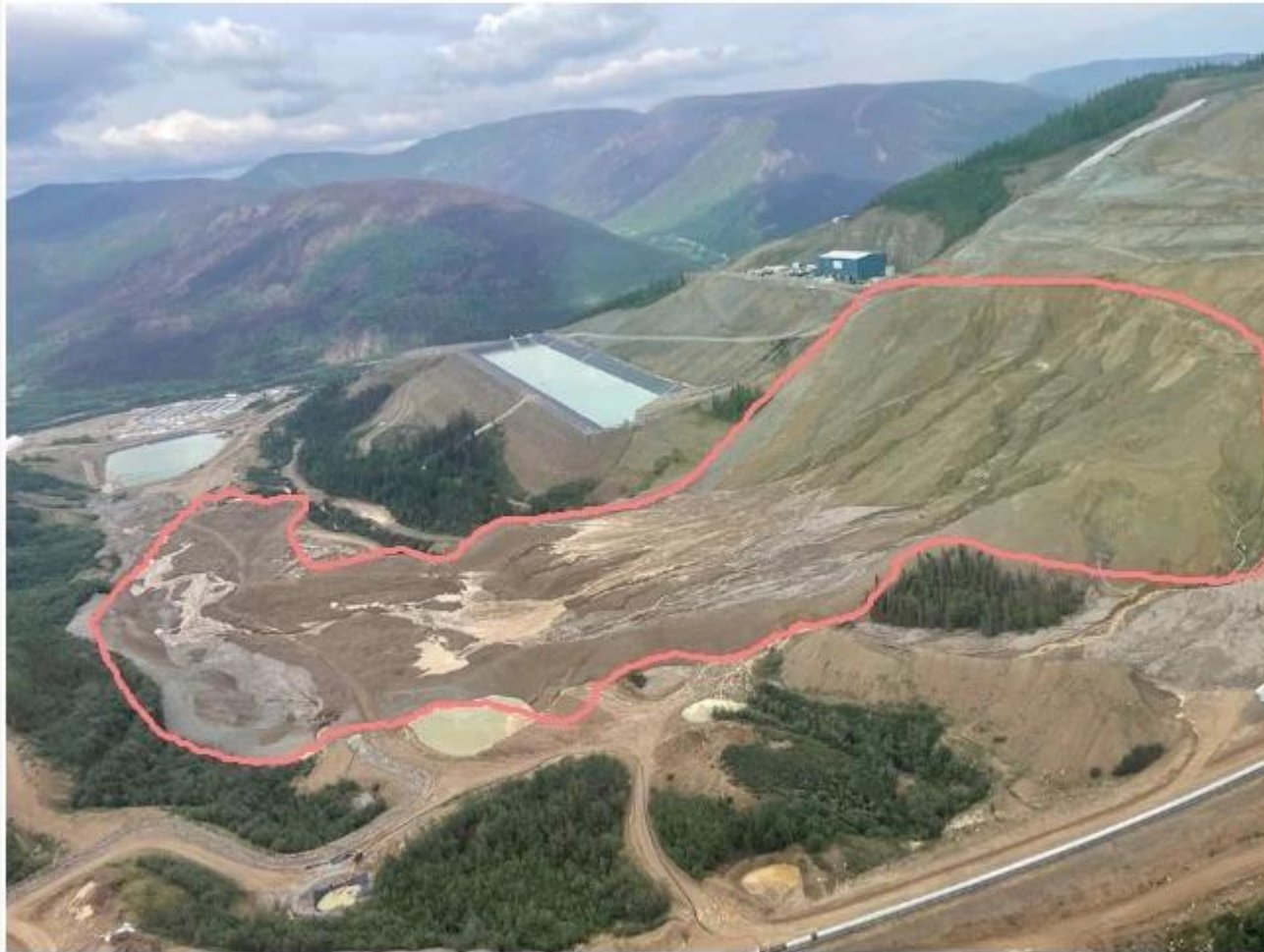
An aerial photo of the landslide off the heap leach facility at the Eagle Gold Mine taken on July 3. (Government of Yukon/Supplied)
