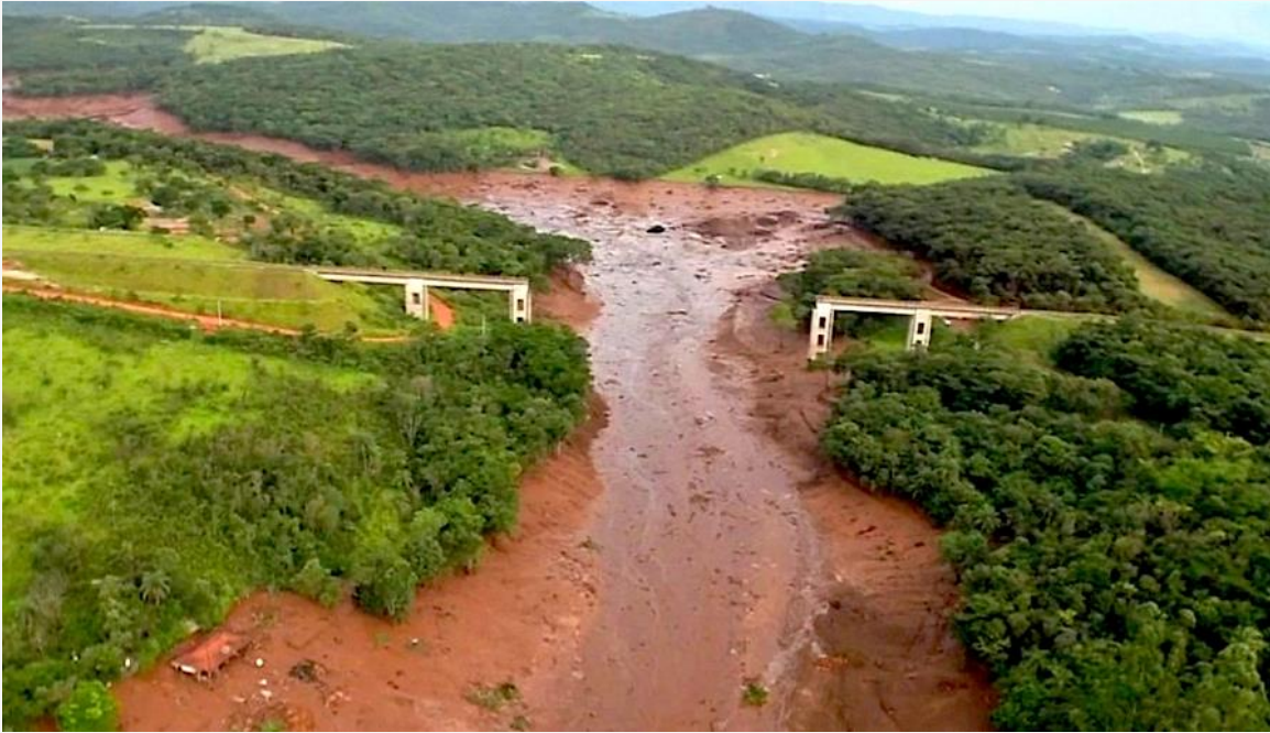
Dam at Brazil Vale's Corrego do Feijão mine that collapsed in January 2019, killing about 270 people. Image: BBC
